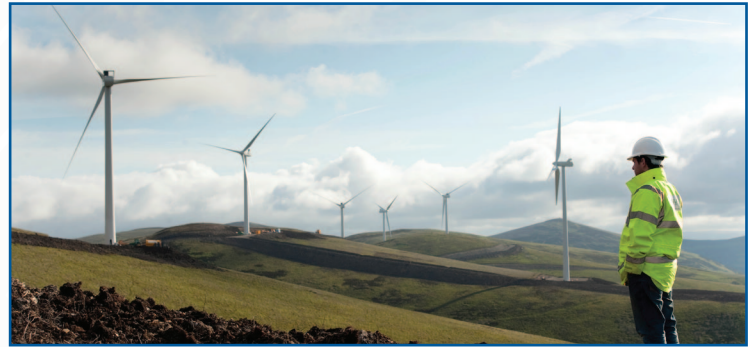
Glenkerie wind farm located on the Scottish Borders. Estimated to prevent the emission of up to 66,000 tonnes of carbon dioxide per year and generate the equivalent of the average annual electricity use of around 16,000 households.
