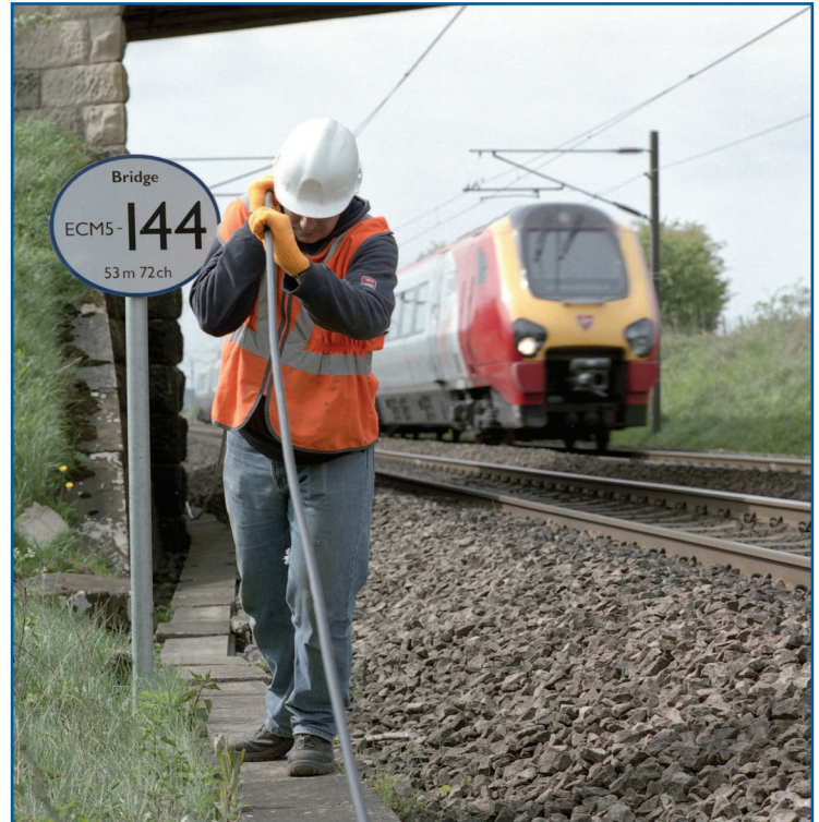
Telecommunications installation by Skanska for Network Rail
