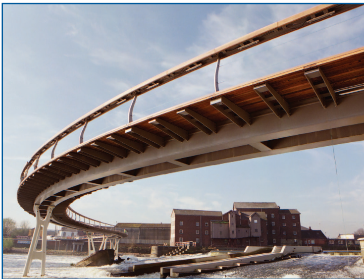
Castleford footbridge - £4.8million landmark structure, is the final and most ambitious of 11 schemes that form 'The Castleford Project', a groundbreaking urban renewal scheme that aims to spark regeneration and a new confidence in this former coal-mining town.
